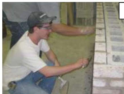
Level 2 Student applying a head joint to a brick
